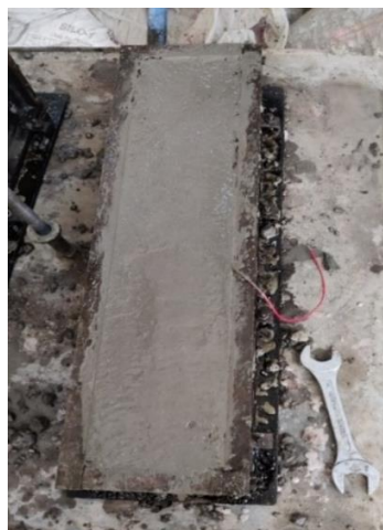
Fig. 3.6 Casting the beams
