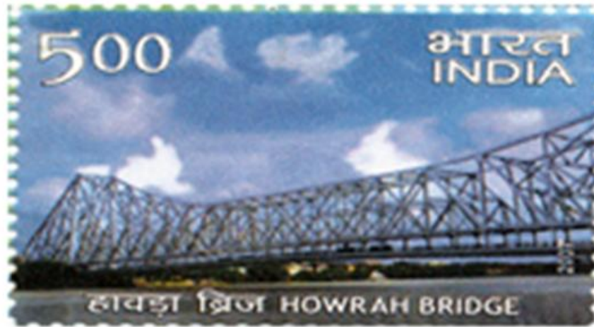
Fig 1.4 View of A commemorative postage on Howrah Bridge [10]
