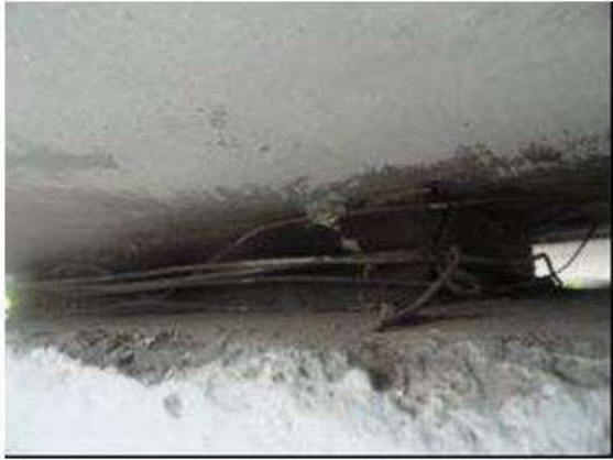
Fig 3.36 MS wire binding around the bearing
