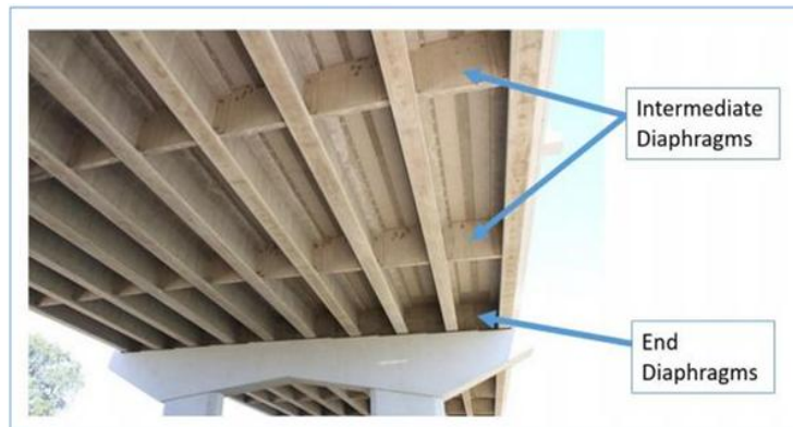
Fig 3.59 Typical view of diaphragms
