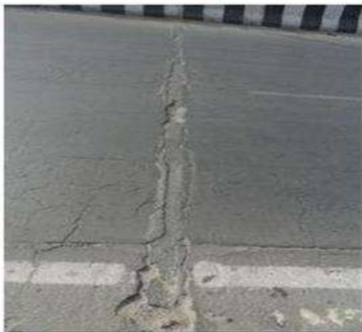
Fig 3.11 wearing course material filled in expansion joint
