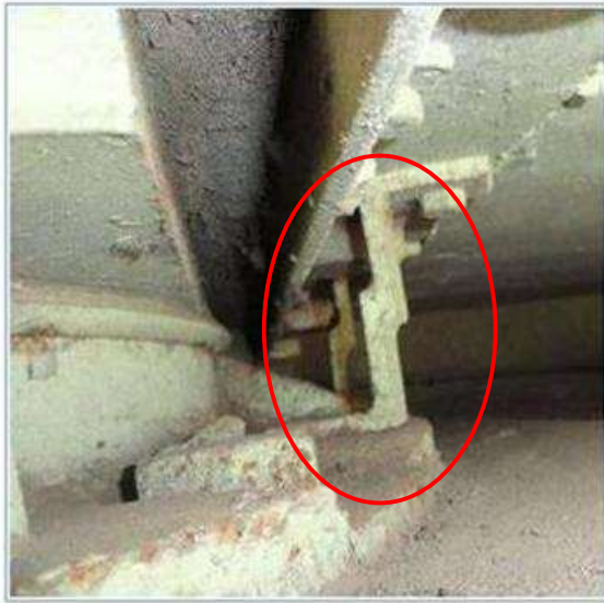
Fig 3.32 Locked bearing is observed as sleeves are not opened for free movement
