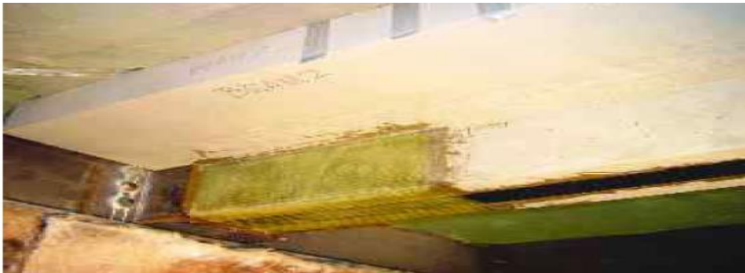
Fig 1.1 strengthening of existing beam with GFRP
