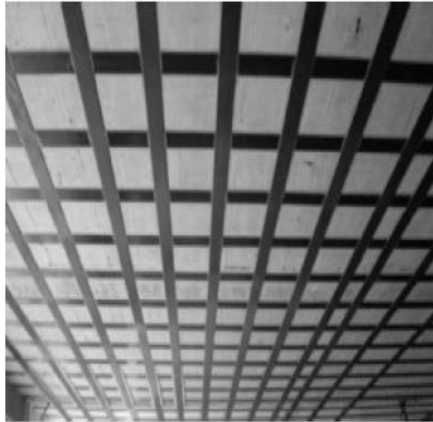
Fig 1.5 Strengthening of existing slab with CFRP
