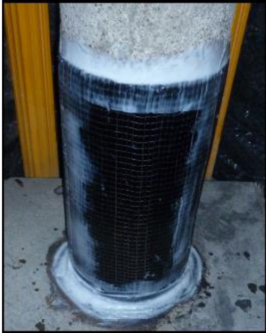
Fig 1.4 Strengthening of existing column with CFRP
