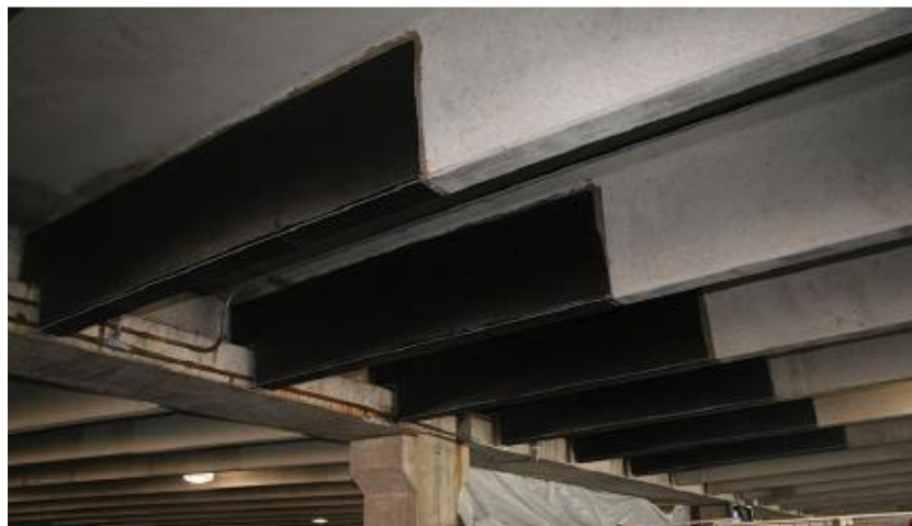
Fig 1.3 Strengthening of existing beam with CFRP
