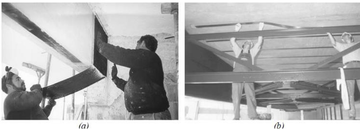
Fig 1.6 Basic FRP application
