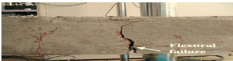
Fig 5.1.Flexural failure of control beam
