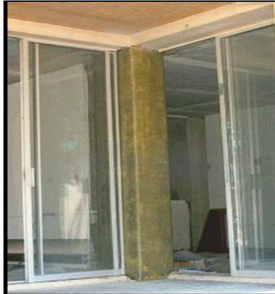
Fig 1.2 strengthening of existing column with GFRP
