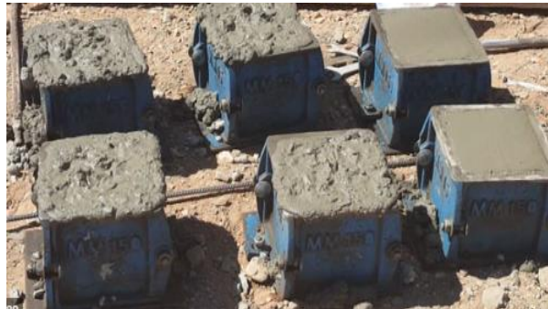
Fig 4.8 . Cubes after casting
