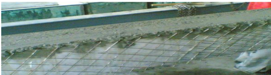
Figure 4.6. Ferro-cement application
