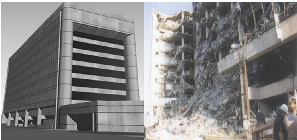
Figure 1.2 Alfred P. Murrah Building before and after the collapse.
