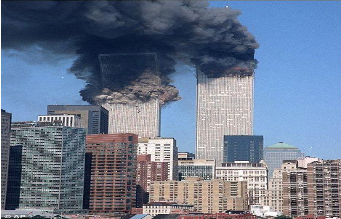
Figure 1.3 Twins Tower, New York (2001)- A case of Progressive Collapse
