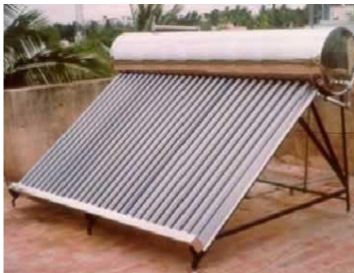
Fig:-1.11 Evacuated tube solar collector
