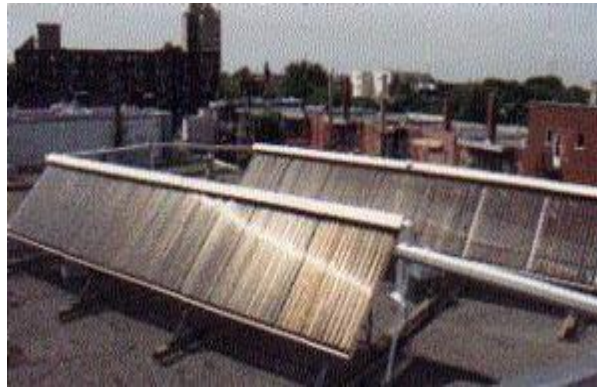
Fig:-1.9 Stationary concentrating solar collectors
