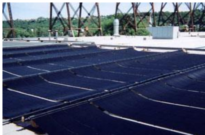
Fig.-1.5 unglazed flat-plate collectors [6]
