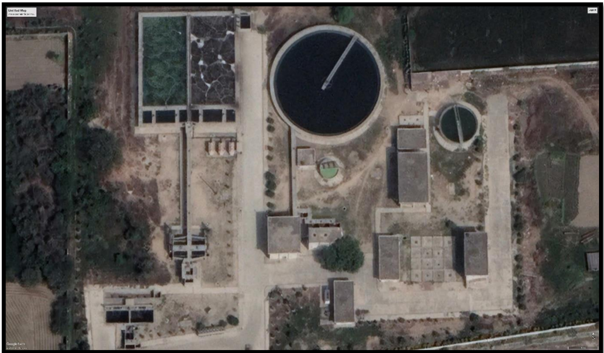
FIG 4.3 SEWAGE TREATMENT PLANT GPS VIEW
