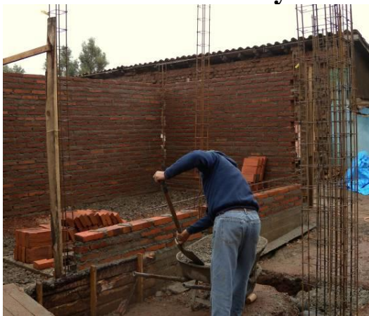
Figure 3: Masonry with infill wall
