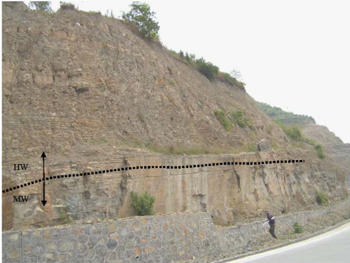
Fig:4 Mechanical and chemical degradation of argillaceous limestone on mountainous slope in three Gorges reservoir, Central China, Zhang Qi (2009).
