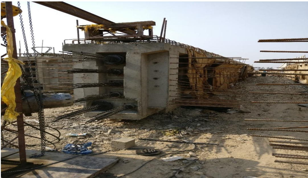
Fig 1.8 Constructed Post-Tension I Girder
