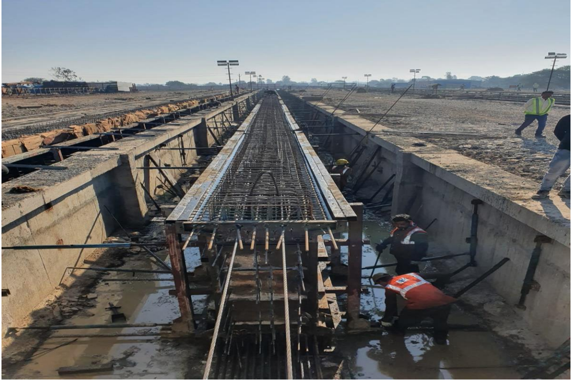
Fig 1.1 Construction of Pretension I Girder in casting bed
