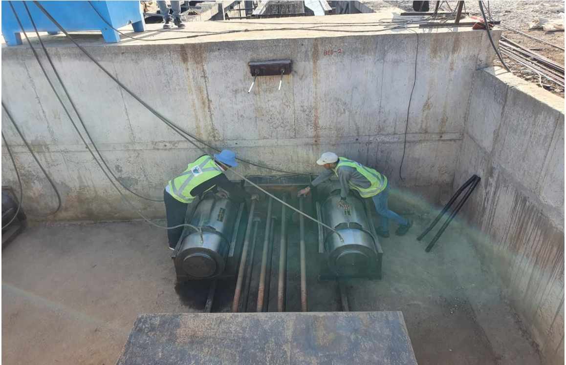
Fig 1.3 Anchor Block Wall & Multi pull jacks of Pretension I Girder
