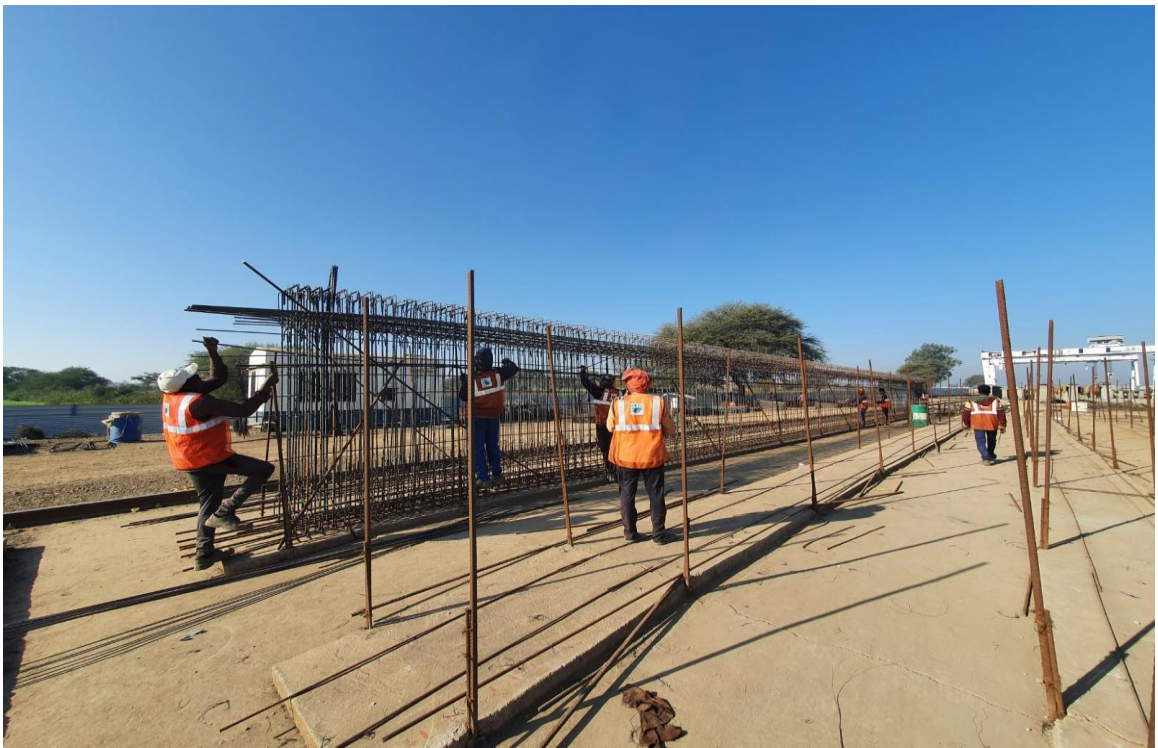
Fig 1.2 Preparation of reinforcement of Pretension I Girder in casting yard
