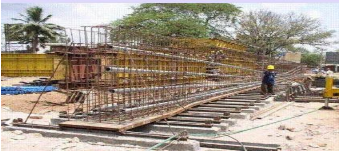
Fig 1.7 Reinforcement Casting of Post-Tension I Girder
