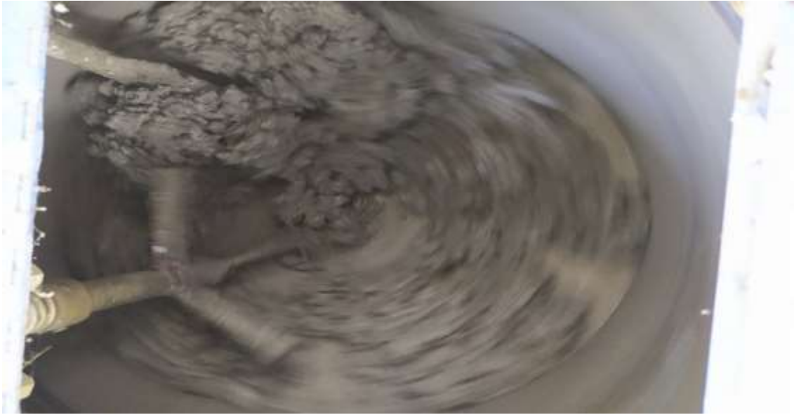
Figure 4.3: Mixing of concrete
