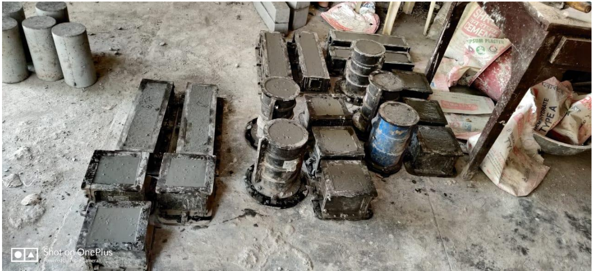
Figure 5.1: Casting of concrete in different moulds.
