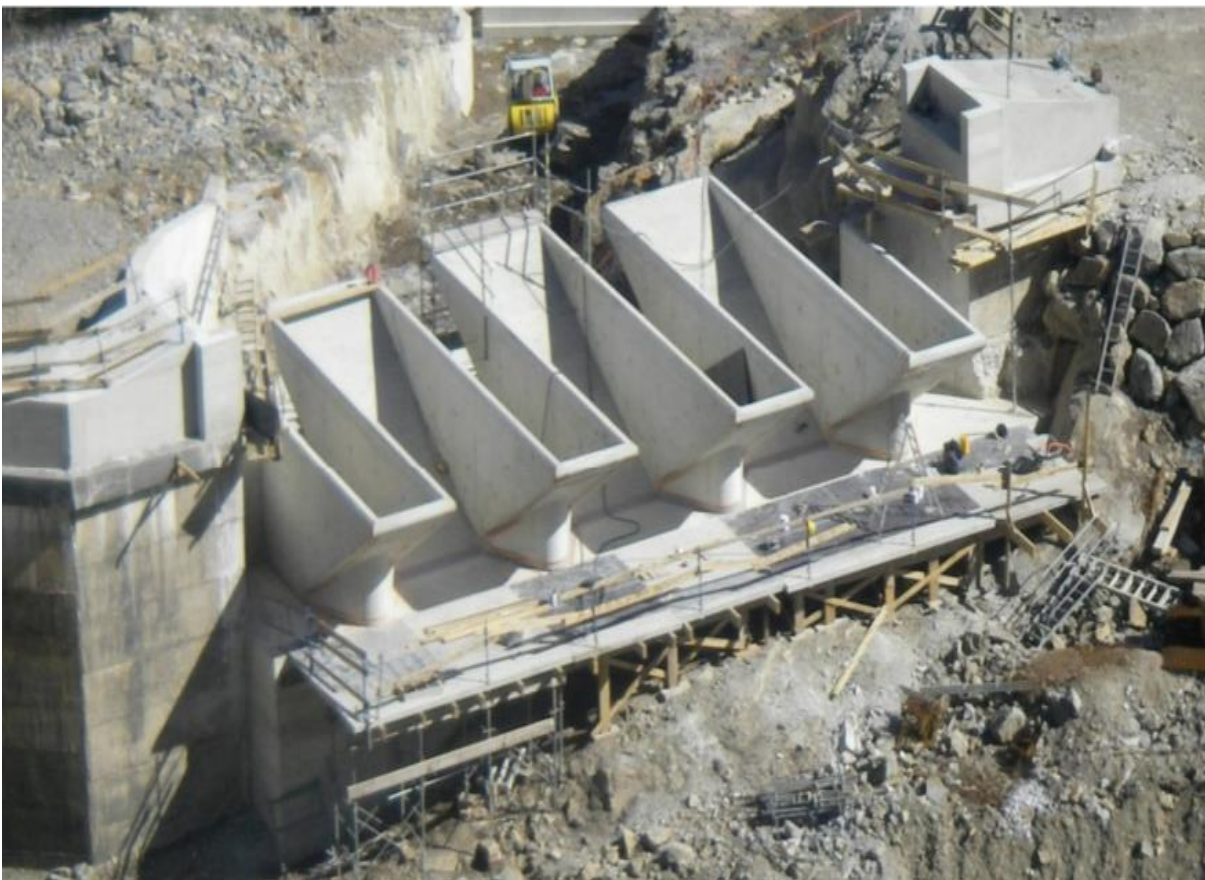
Fig-1.6 Diagram showing Piano key Weir.
