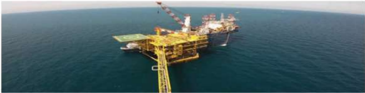
A fully-integrated gas platform - the heaviest in Saudi Aramco's history - installed by float-over method at Hassbah FMS in Saudi Arabia
