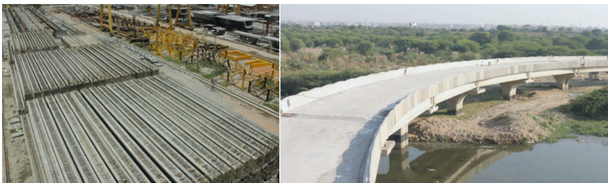
Fig. 52: Precast Pre-tensioned beams stacked in casting yard
