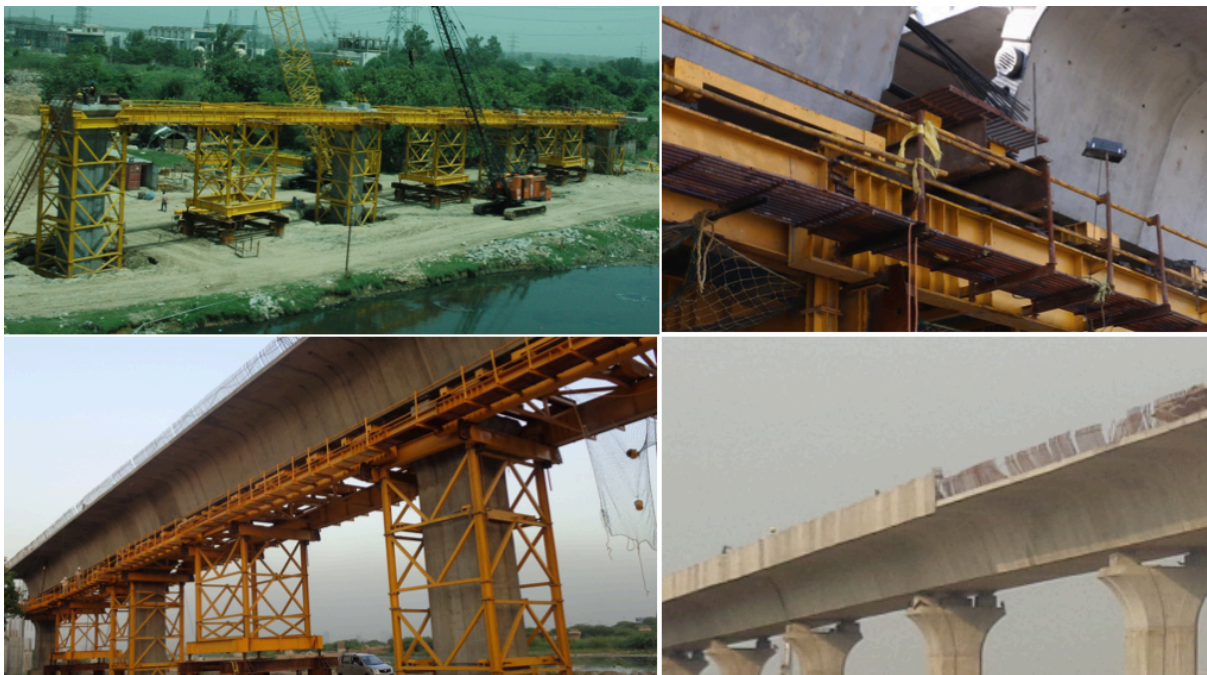
Fig. 50: Ground launching of spans making it continuous
