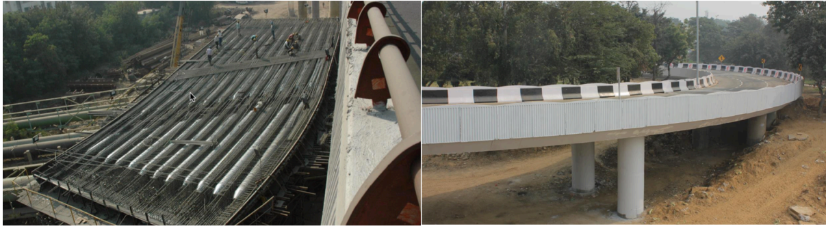
Fig. 56: Voided slab monolithic over circular piers
