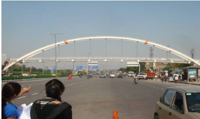
Fig. 24: Pedestrian foot-over bridge
