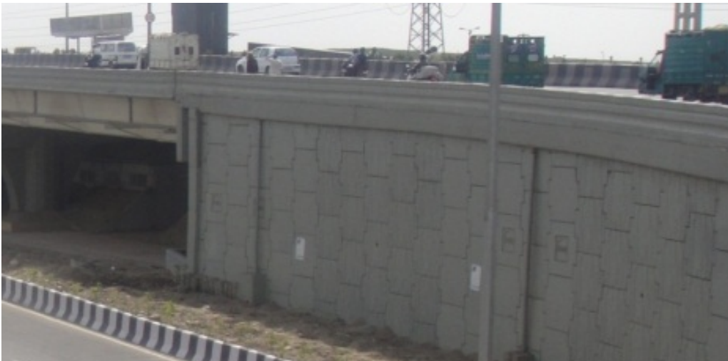
Fig. 27: Reinforced earth wall
