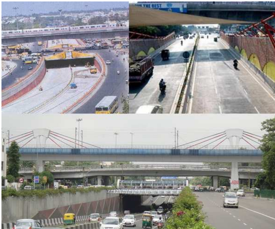
Fig. 12: Underpasses constructed in new millennium
