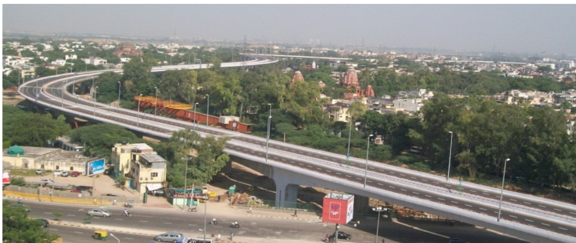
Fig. 15: Barapullah elevated corridor (in Phase 1)
