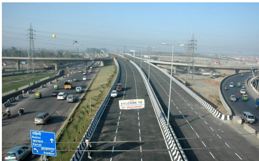
Fig. 19: A view of Mukarba Chowk grade separator
