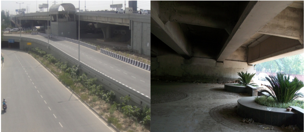
Fig. 28: Greenery in area outside as well as under the viaduct
