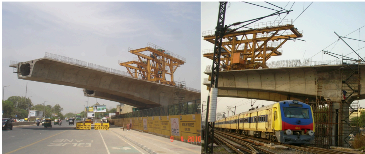
Fig. 23: Road and rail traffic continued during construction
