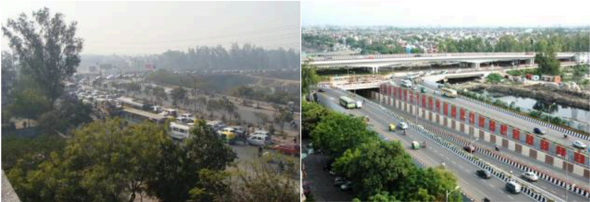
Fig. 25: Ghazipur crossing before and after construction
