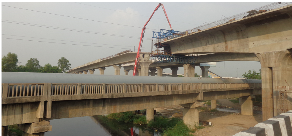
Fig. 51: Cantilever construction for long spans
