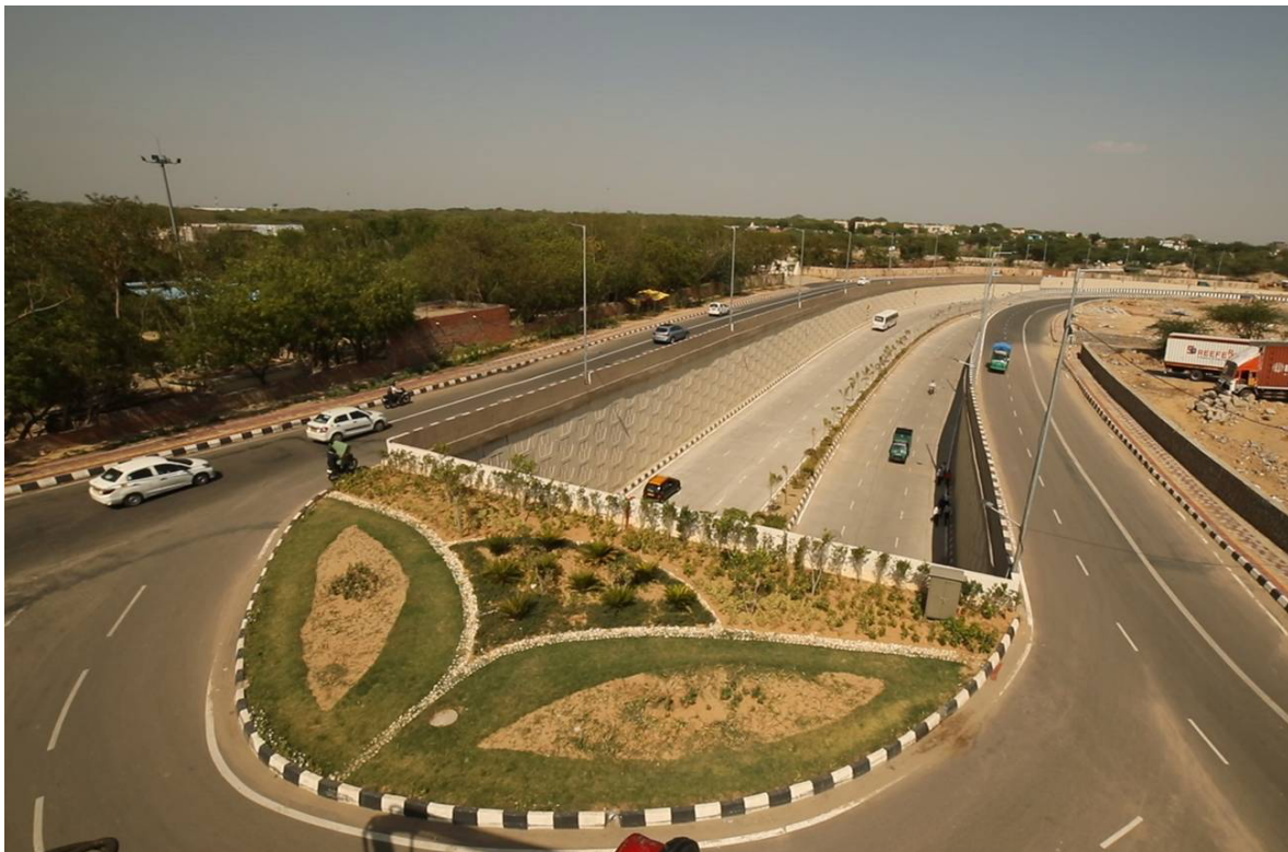
Fig. 18: Mahipalpur project with two flyovers and an underpass
