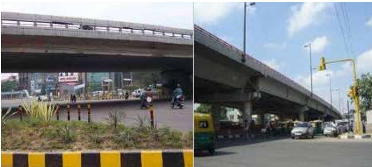
Fig. 8: Flyovers with Precast Pre-tensioned RCC beams
