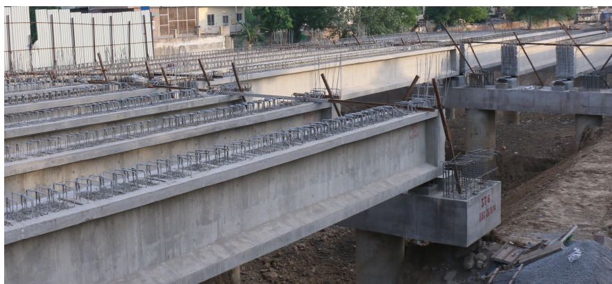
Fig. 53: Pre-tensioned beams for structure over nallah
