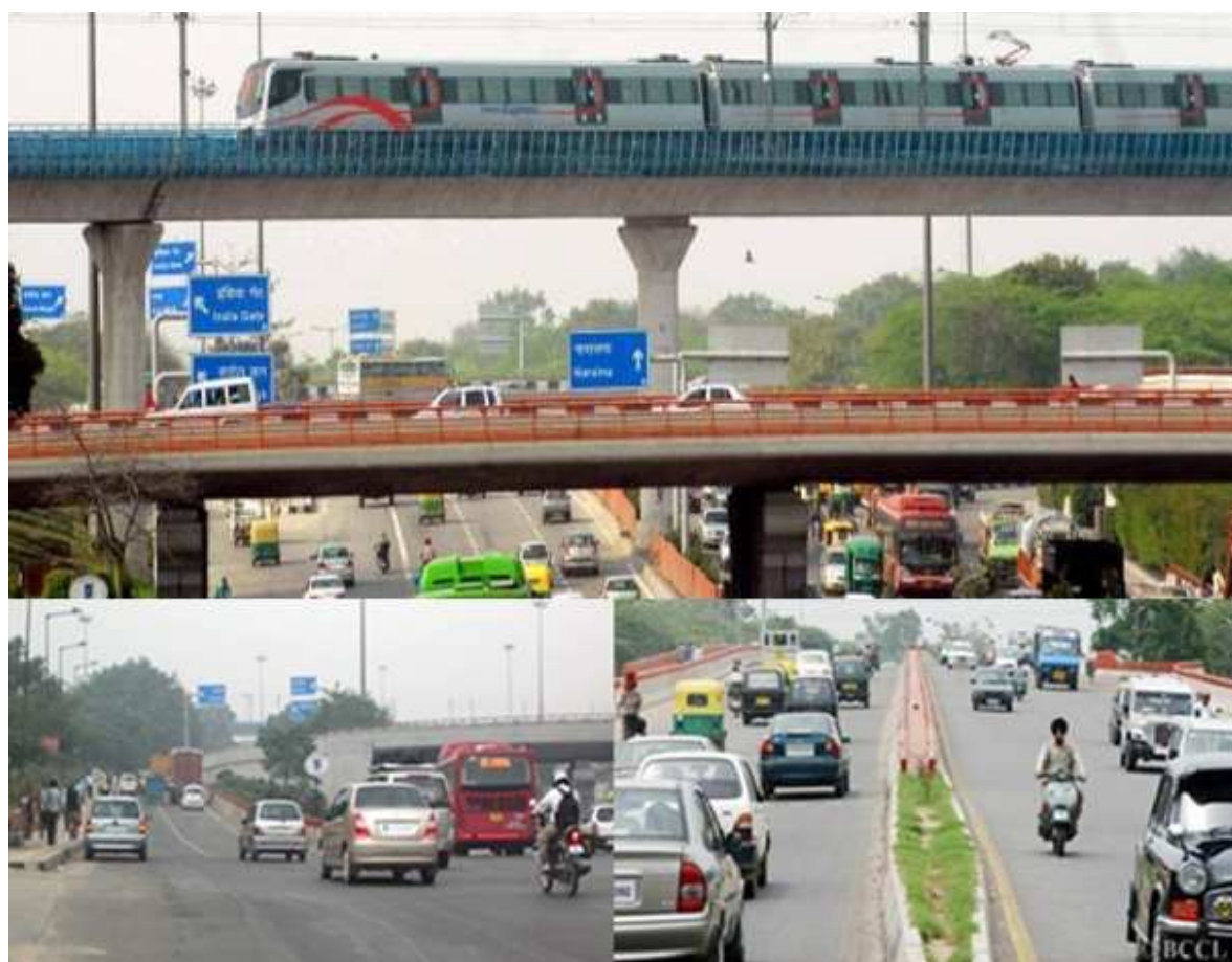
Fig. 10: Grade separator at Dhaula Kuan (5 arms)
