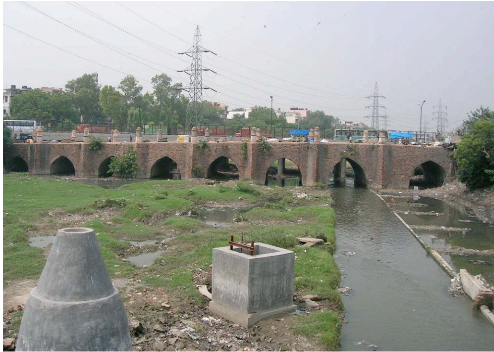
Fig. 21: Barapullah Nallah: 12 bridges in view
