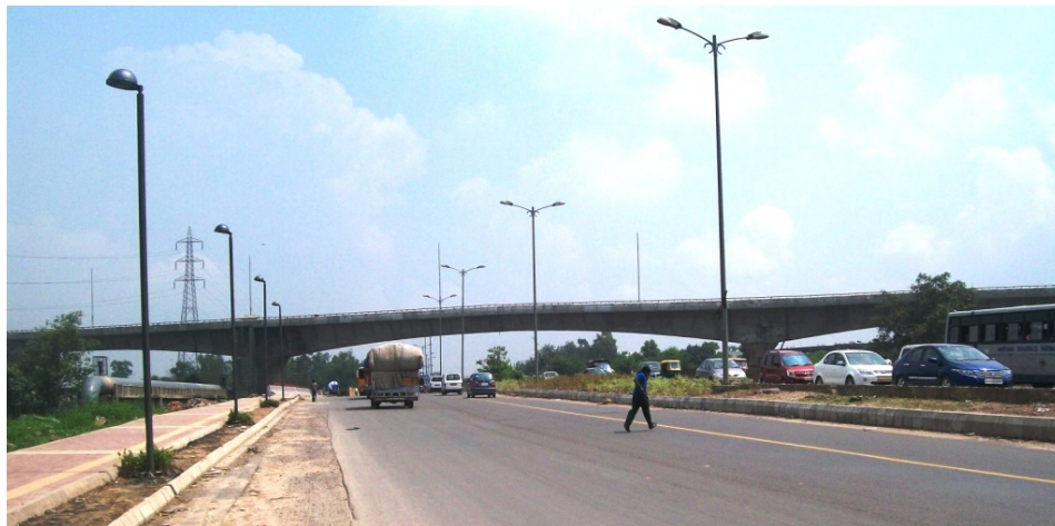
Fig. 26: Longer spans to cross the major road
