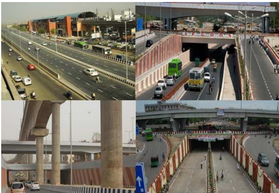
Fig. 14: Flyovers with 3 level grade-separators
