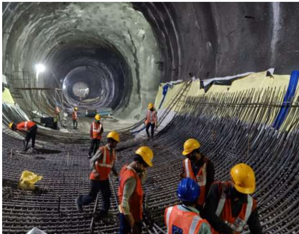
Figure 6: Tunnel after TBM excavation (Mumbai Metro line-3)
