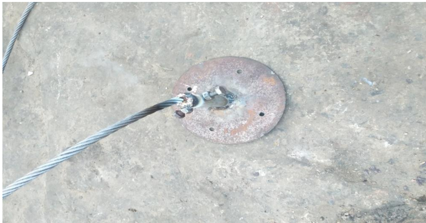
Fig.3.10 wire rope welded with circular plate
