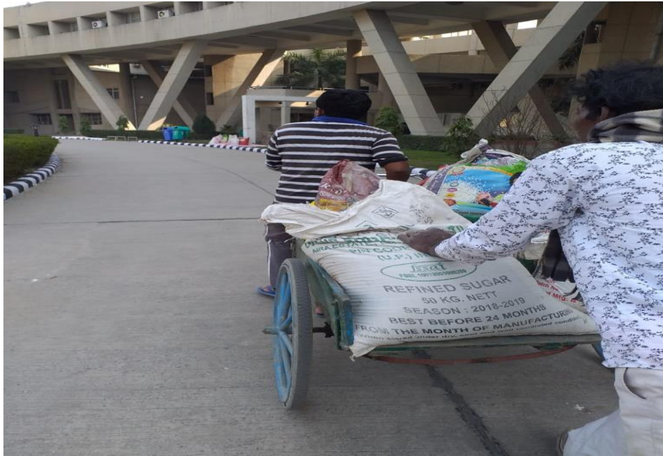
Fig. 3.1 Transporting sand bags at site
