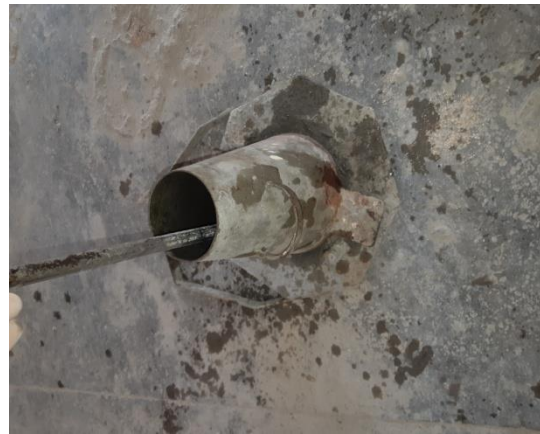
FIG-33[ After filling 1/4 th and tamping with rod]
