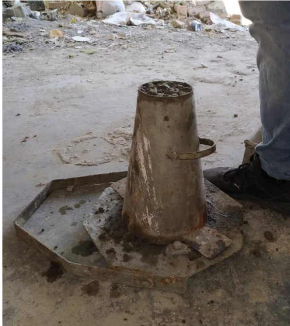
FIG-34 [ Concrete filled to the top ]
