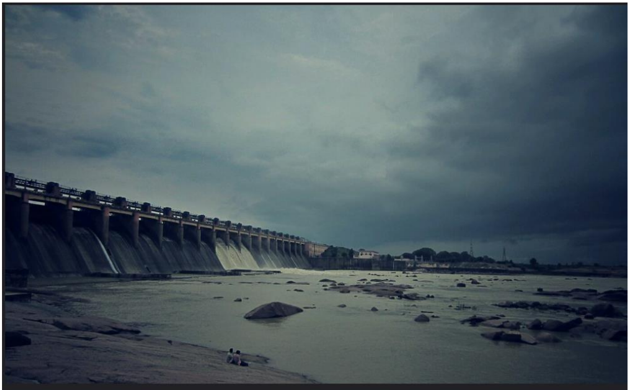
Fig. 6 – Matatila dam at a glance
