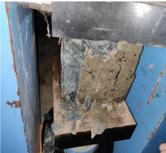
Figure 4.5 Failed under compression
