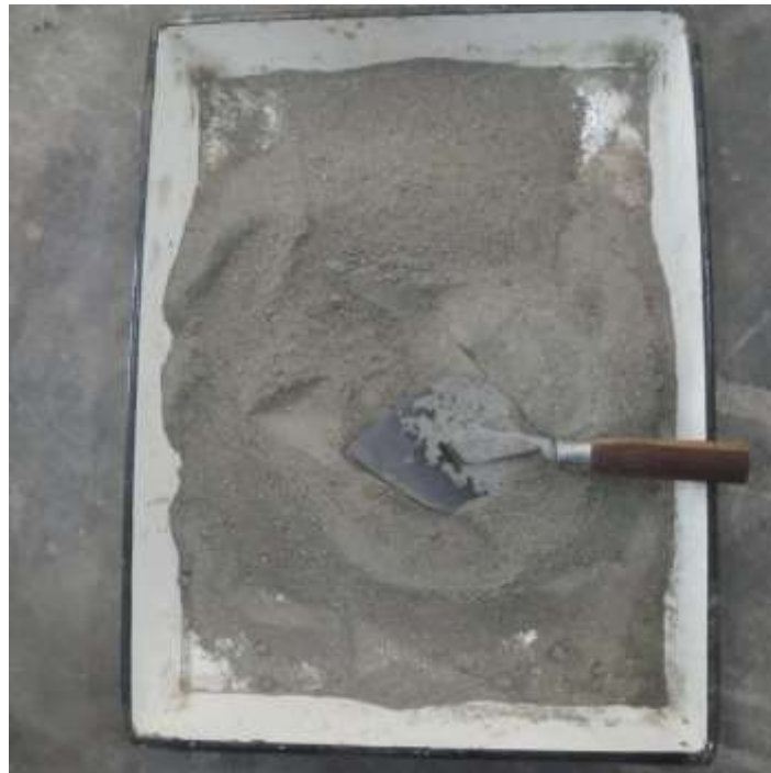
FIG 3.5 - Mixture of cement and sand in dry state
