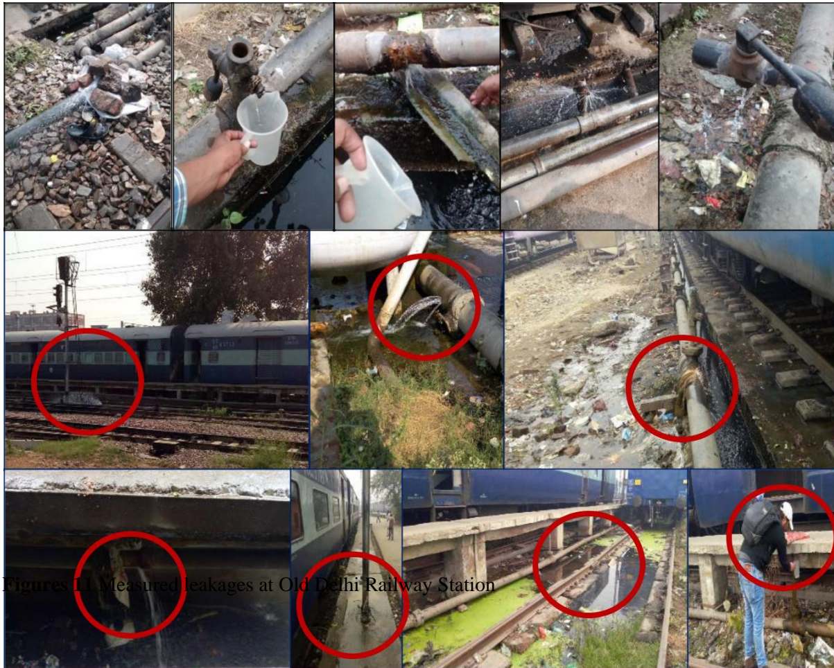
Figure 15 Leakages points at Station
