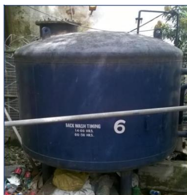
Figure 5 Rapid Sand Filter
