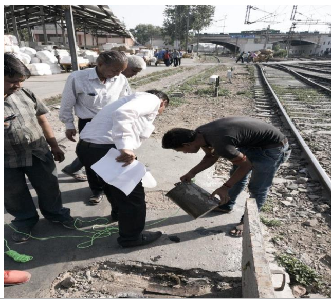
Fig.10: Extracted Sewage sample from Manhole
