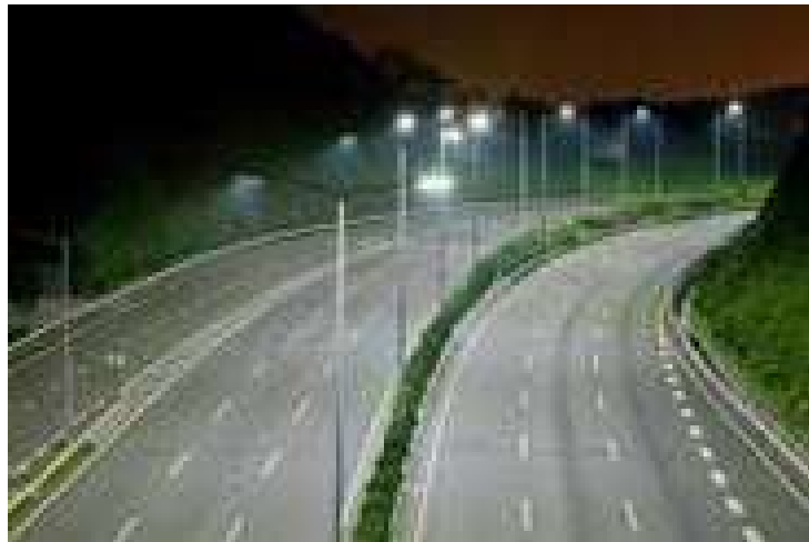
Figure 4: Typical highway lighting view
