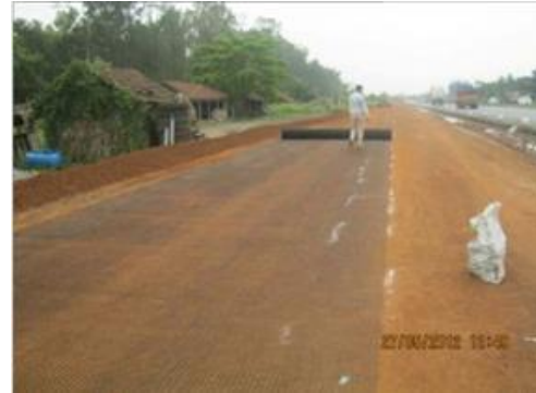
(b) Laying down of geogrid in pavement
