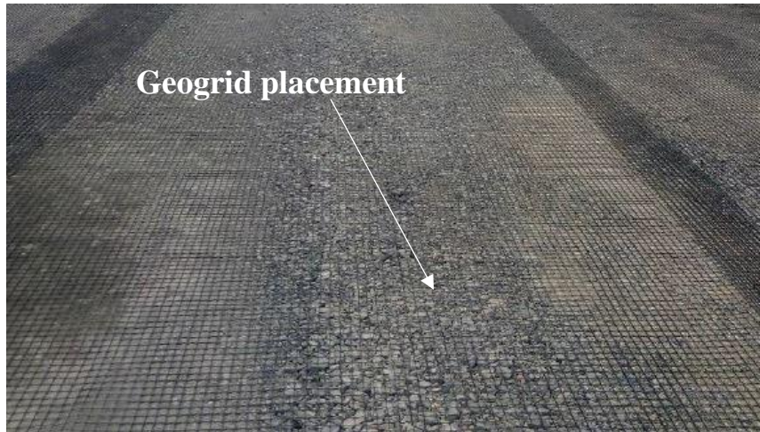
Fig. 1.4 Laying down of geogrid in granular sub base (HMBS Textile, 2017)
