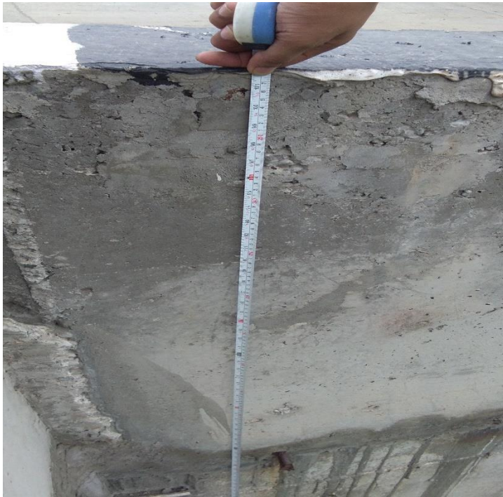
Fig 8: Measurement of height of front wall
