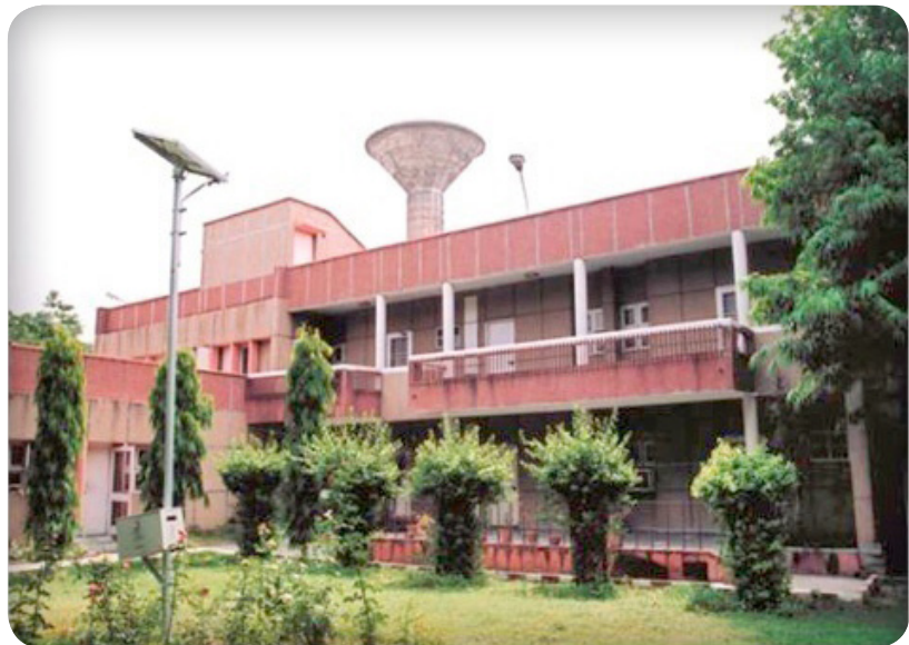
Guest House (8 Double Bedded Rooms)
