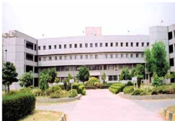
Mechanical Engineering Block
