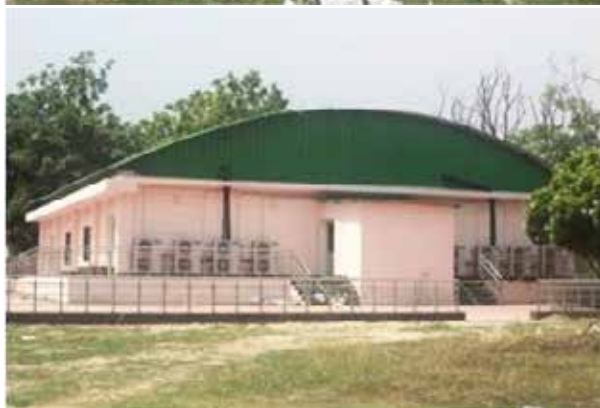
Construction of 2 Nos. Lecture Halls (IIT Pattern)
