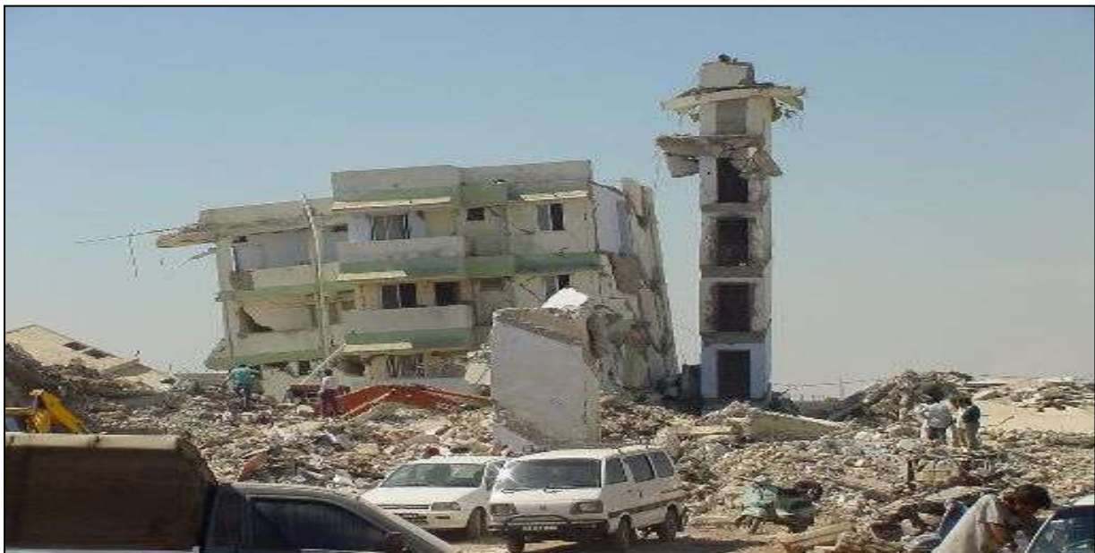
Figure 3.1 Damaged building in Gujrat Earthquake 2001
