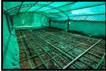
Figure 4.14 Wastewater distribution over Bio-filter bed.
