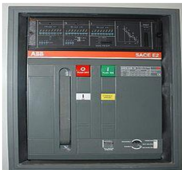
Figure 4: ABB SACE E2 1250A Air Circuit Breaker of ABB.
