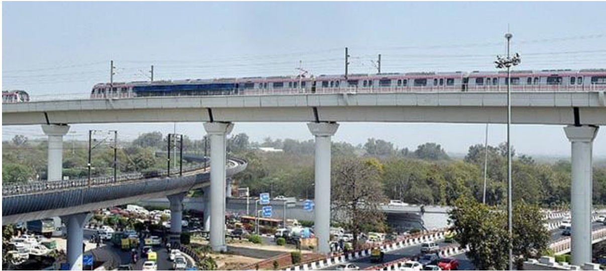
Figure 1.2 Box Girder Bridge,DMRC,Delhi
