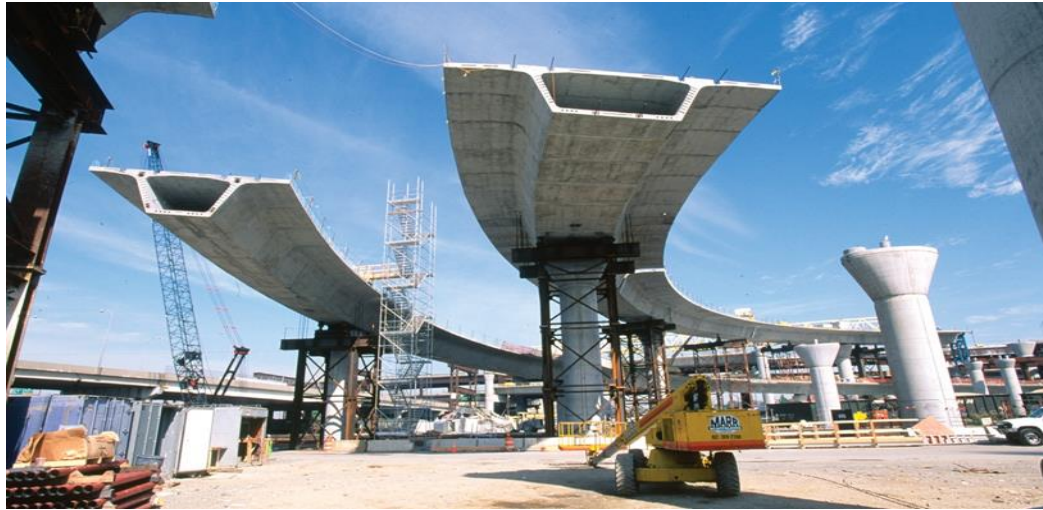
Figure 1.1 Image showing Bridge of Box Girder type
