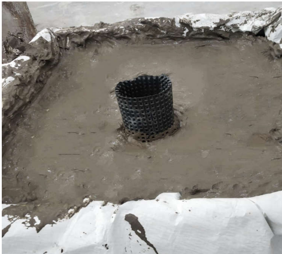
Fig. 3.12. Granular column encased with geotextile
