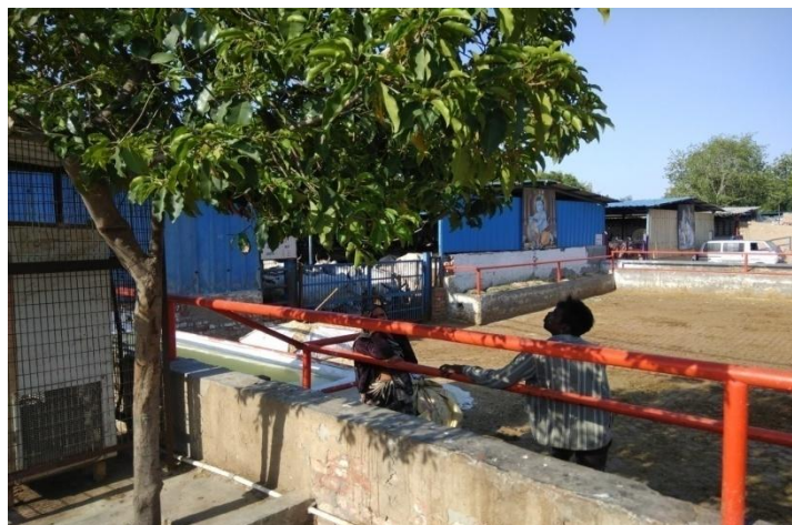
Figure 8.5: Shri Krishna Gaushala Cow Shed
