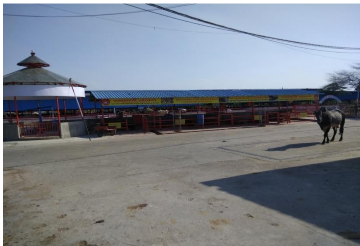
Figure 8.4: Shri Krishna Gaushala Cow Shed
