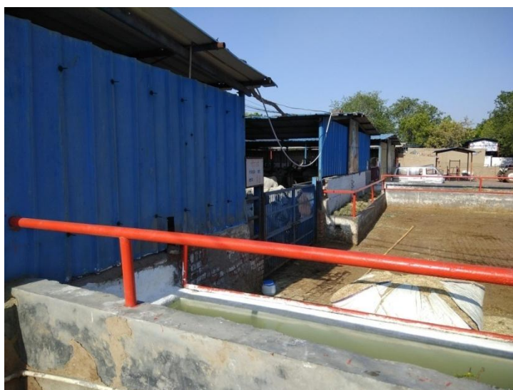
Figure 8.6: Shri Krishna Gaushala Cow Shed
