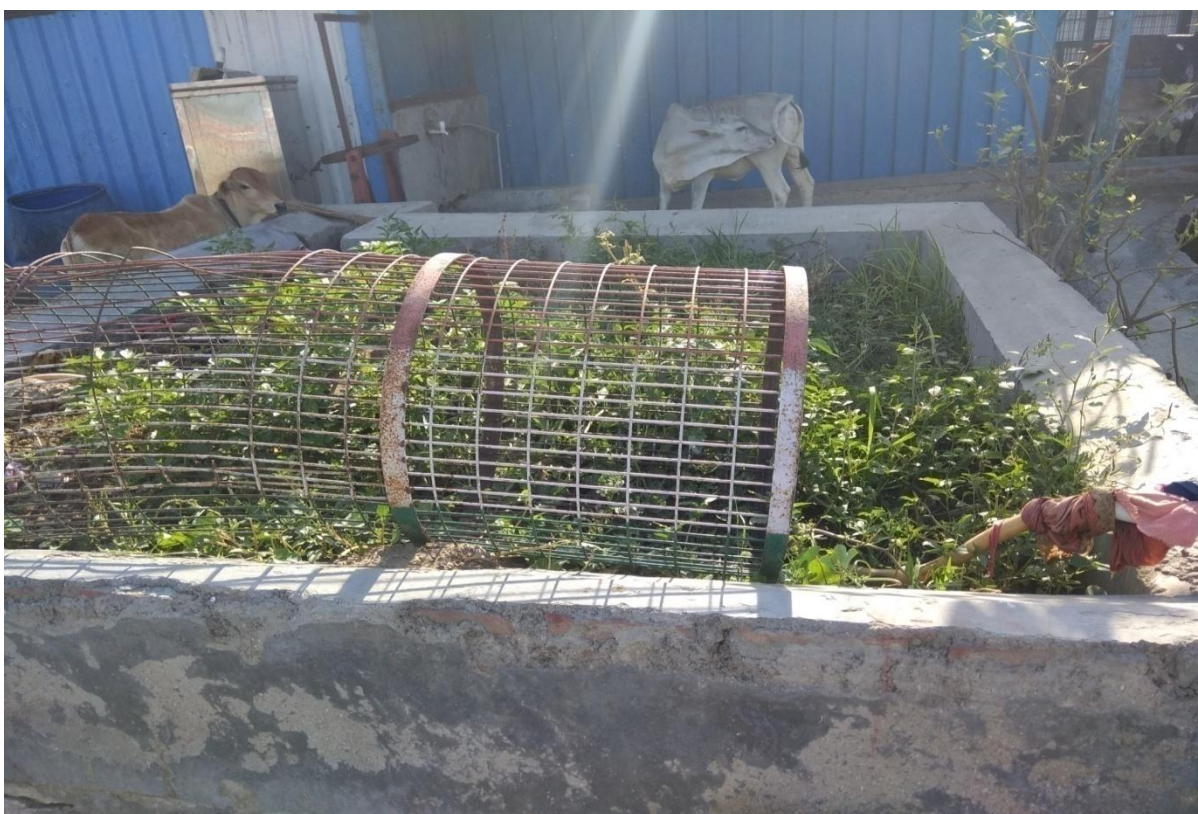
Figure 8.8: Shri Krishna Gaushala Biogas Plant Slurry Outlet
