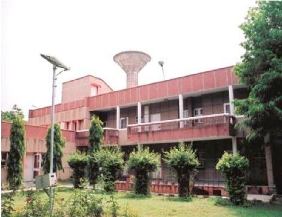
Guest House (8 Double Bedded Rooms)
