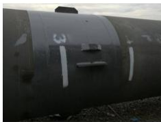
e) steel pipe pile caisson
