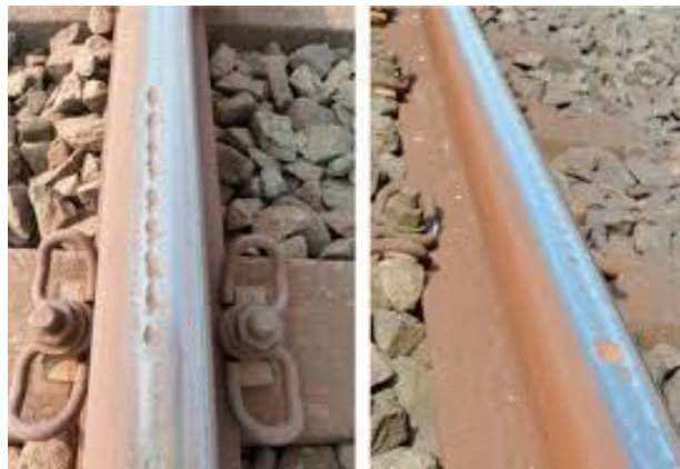
Fig.1.6: Chipping of material from the side and top surfaces respectively
