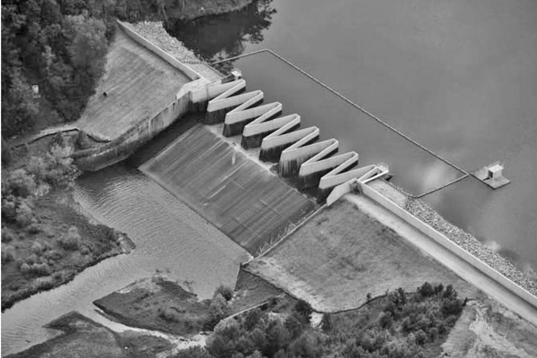
Fig. 2.1 Raised labyrinth shape spillway at Dog River Dam, Georgia [1]
