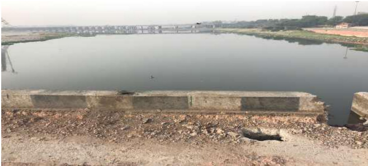
FIGURE 3.1 SAMPLING LOCATION AT WAZIRABAD BRIDGE
