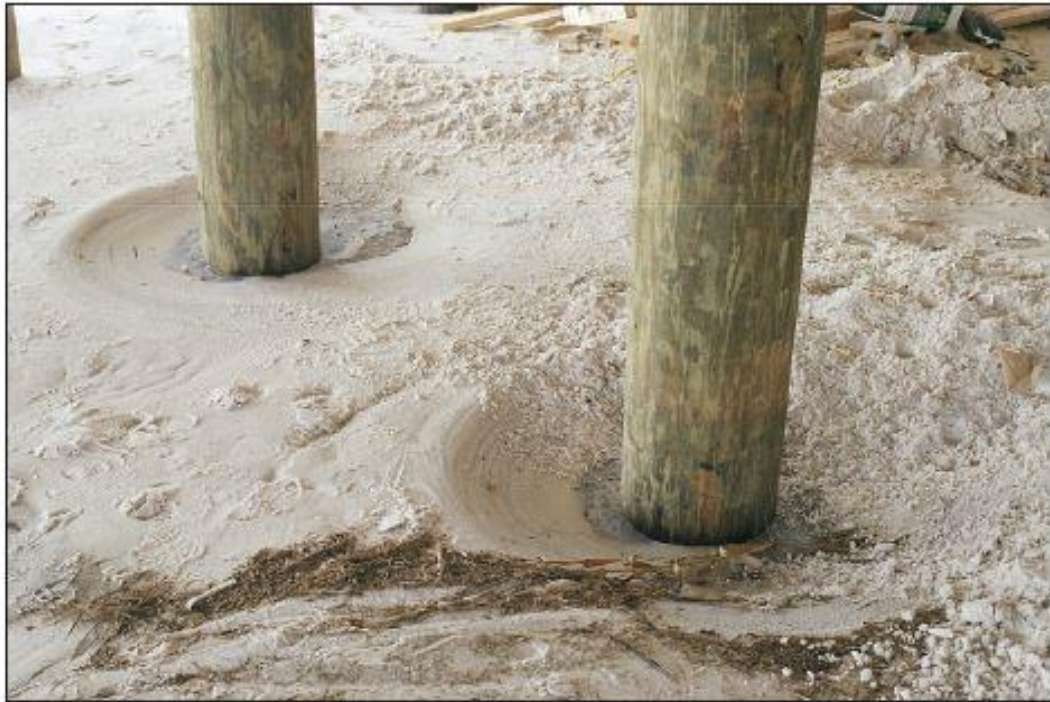
Figure.1.5 Sketch showing the local scour (Source: Erosion, Scour and Foundation Design, FEMA,2009)
