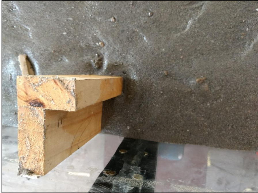
Figure.4.13 Scour formation around LU-3
