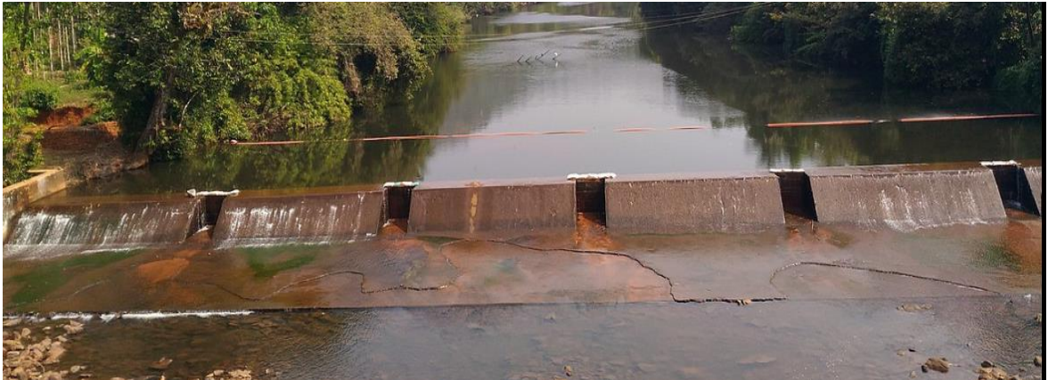
Figure 1.12: Check dam at Kudumboor across Chandragiri River.
