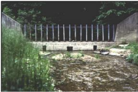
Figure 1.14: Screen dam and vertical bars for retention of mainly vegetative materials.
