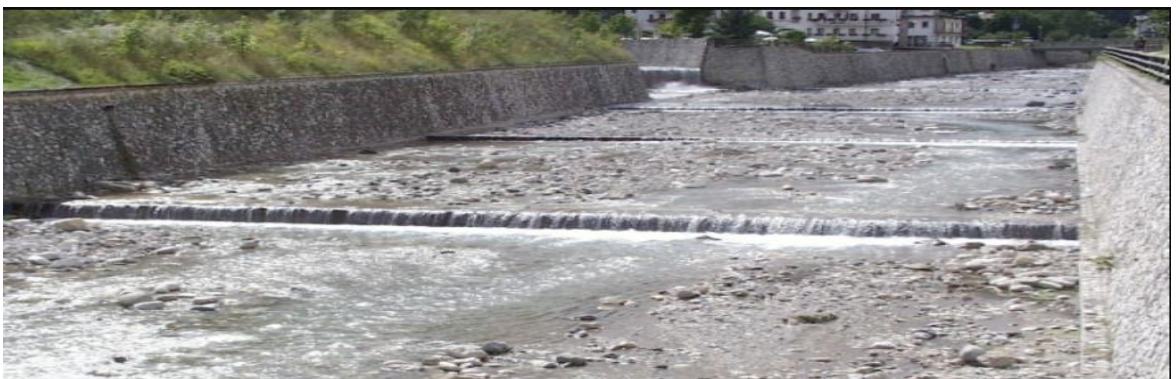
Figure 1.13: Low height bed sills.
