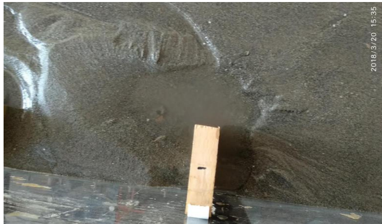
Figure 5.8.1: Scouring around first short length impermeable groyne.
