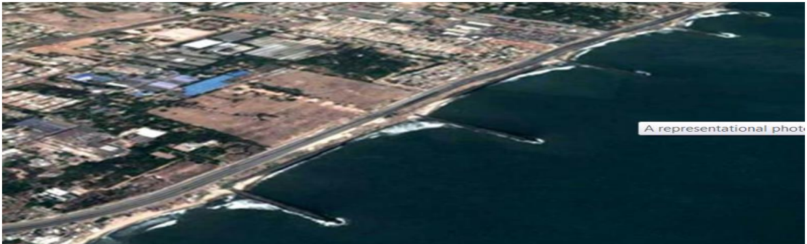
Figure 1.16: Transverse groynes laid in Kerala beach by IIT-Madras (2007).
