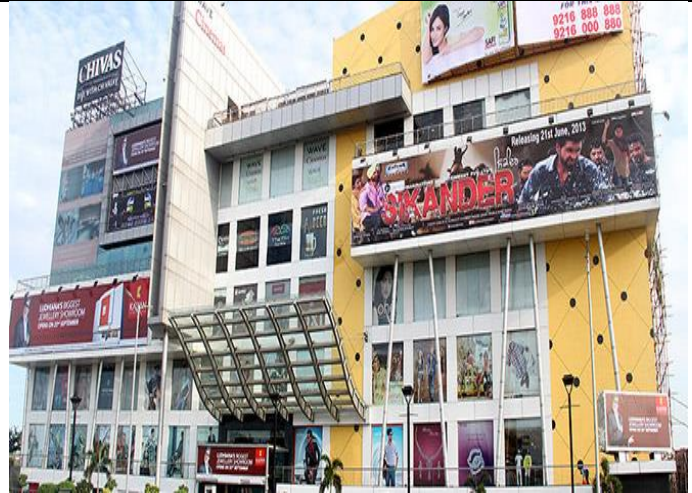
Structure 25- Waves Mall
