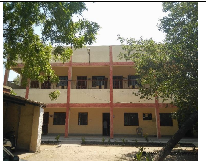
Structure 29- AXEN C office
