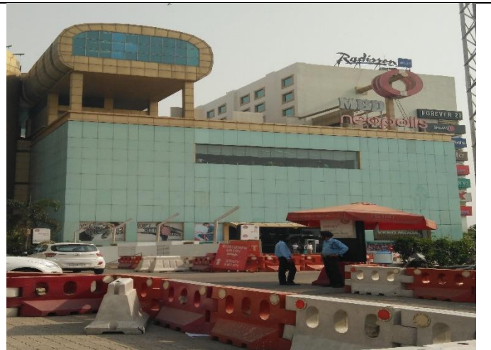
Structure 27- MBD Neopolis
