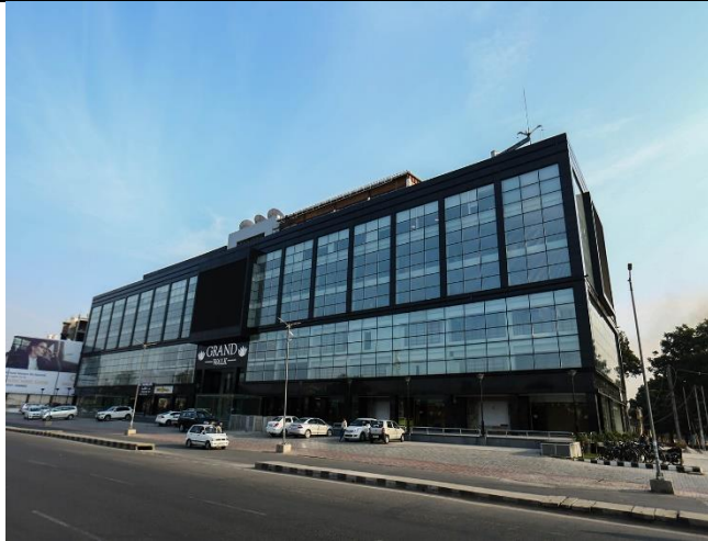
Structure 24- Grand walk mall
