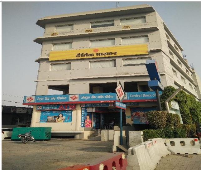
Structure 28- Dainik Bhaskar Office
