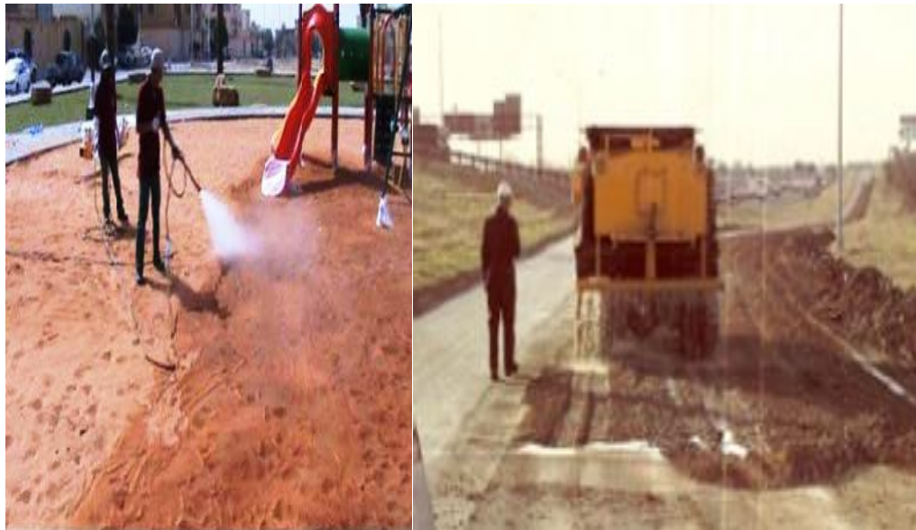
Fig.2.2 Chemical stabilisation of soil
