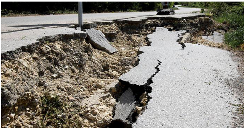
Fig 1.4 Failure-of-pavements-on-collapsible-soil
