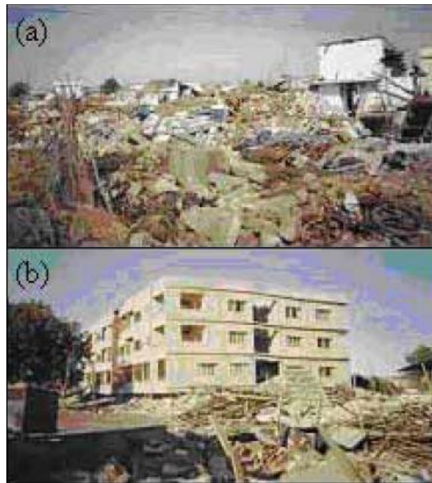
Fig1.2 (a) Ratnal Village was destroyed due to bhuj earthquake and (b) Ground Floor of RC building was collapsed in Bachau ( iitk.ac.in )
