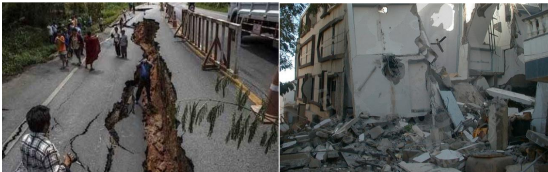
Fig1.3: left image-crack in road due to bhuj earthquake ( newsnation.com ) and right image building collapse in bhuj earthquake ( civildigital.com )
