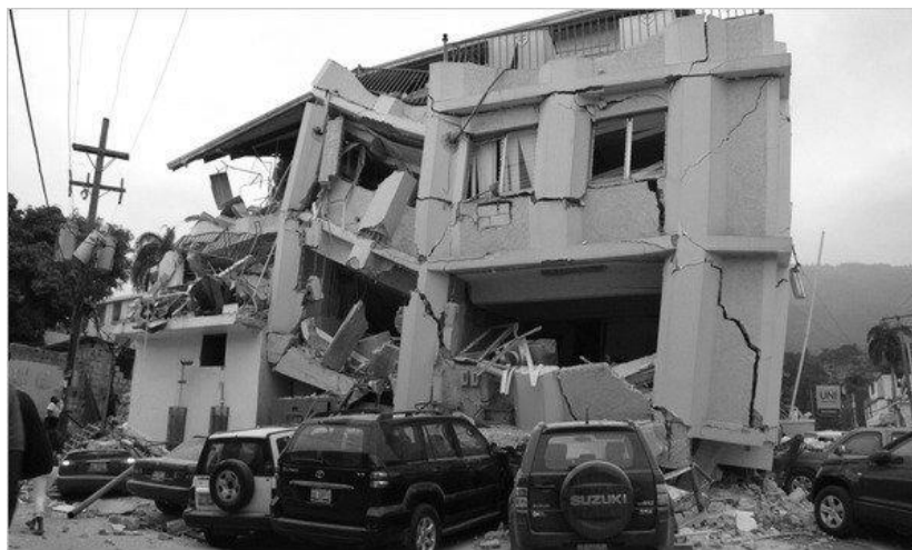
Figure1.1: Failure of unreinforced masonry
