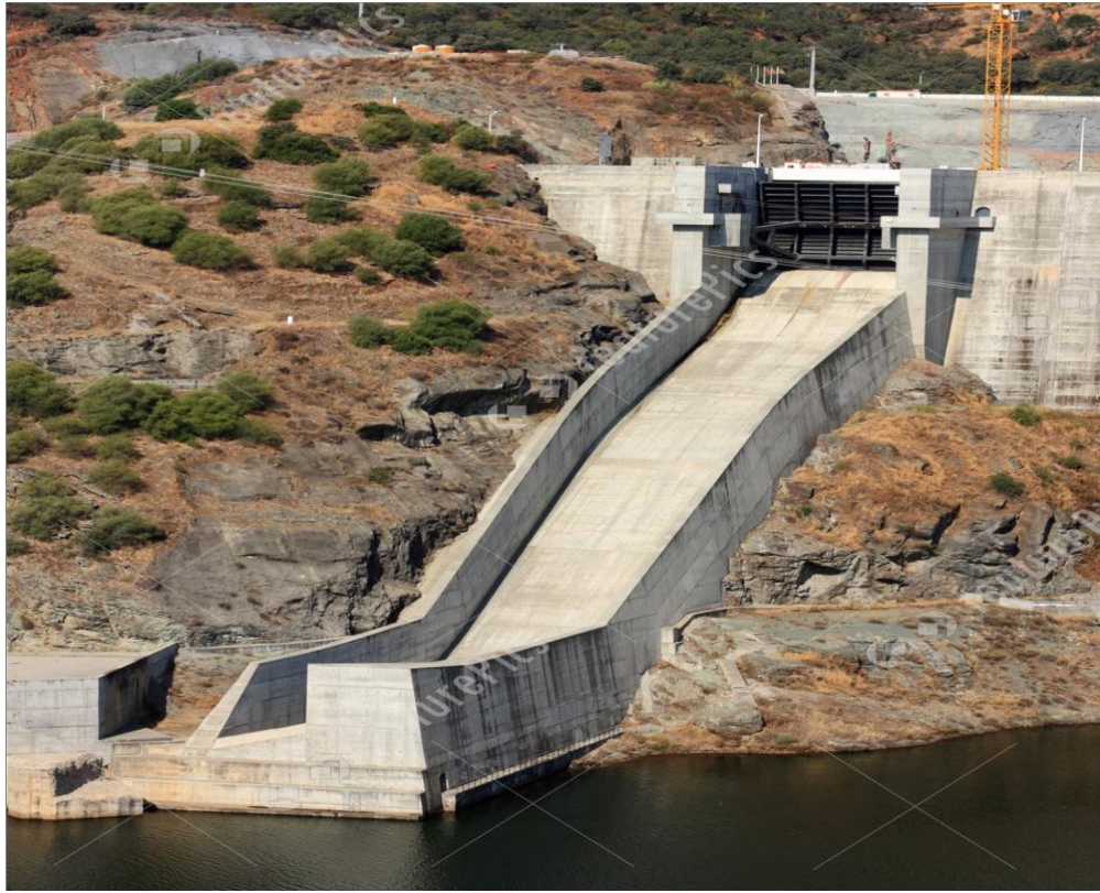
Figure 1.5 Alqueva dam chute spillway, Portugal
