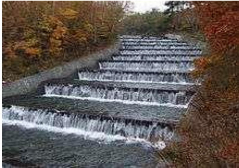
Fig 1.11 stepped or cascade spillway
