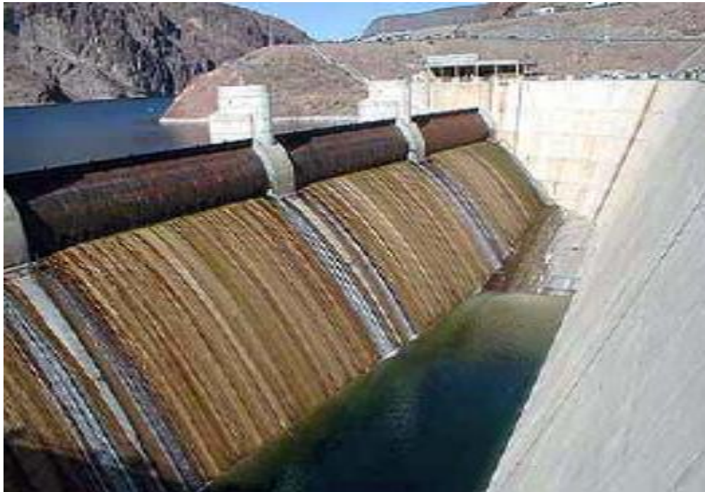
Figure 1.6 Hoover dam, USA
