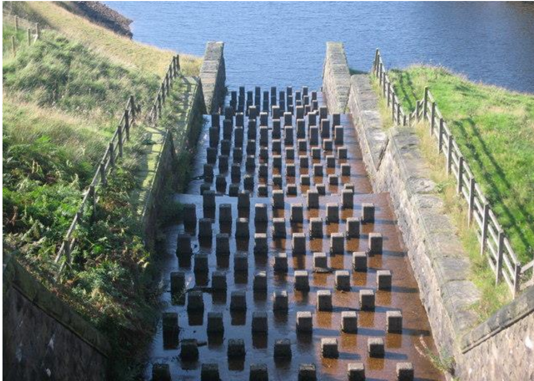
Fig 1.11 Baffle chute spillway
