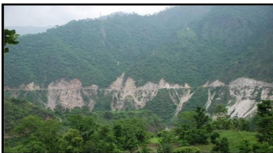
Fig. 1.2: Jhakri slope failure along NH-5 (Source: HPSDMP Himachal Pradesh) (Link: hpsdma.nic.in/DisasterManagement/HPSDMP.pdf )
