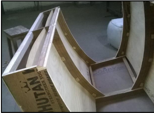
Fig. 3.4 Wooden cradle backed by supporting frame
