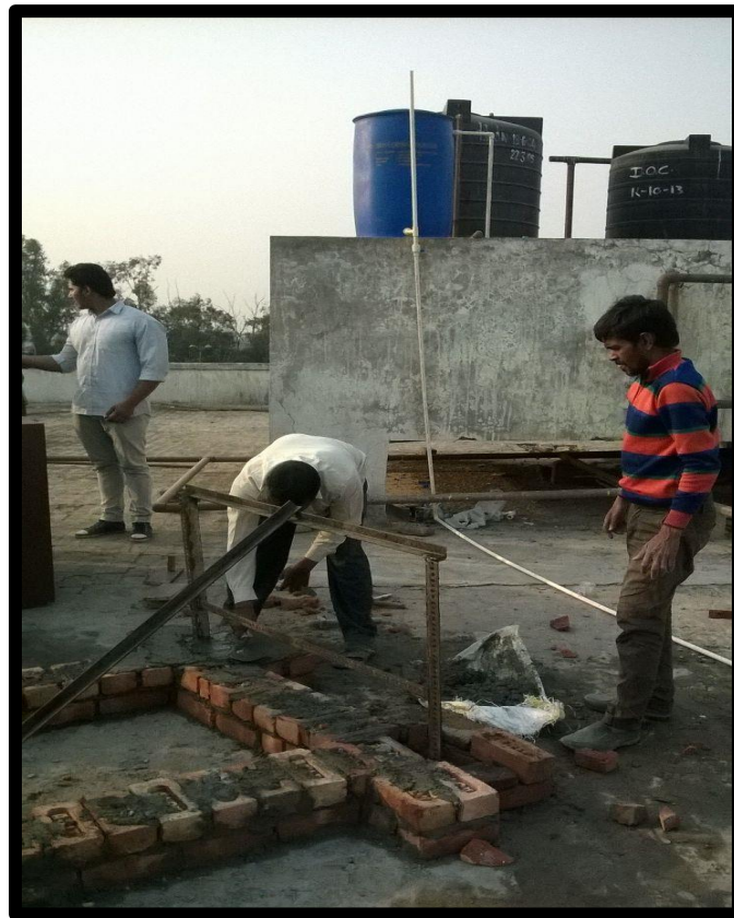
Fig 3.19 Masonry work for roof top installation
