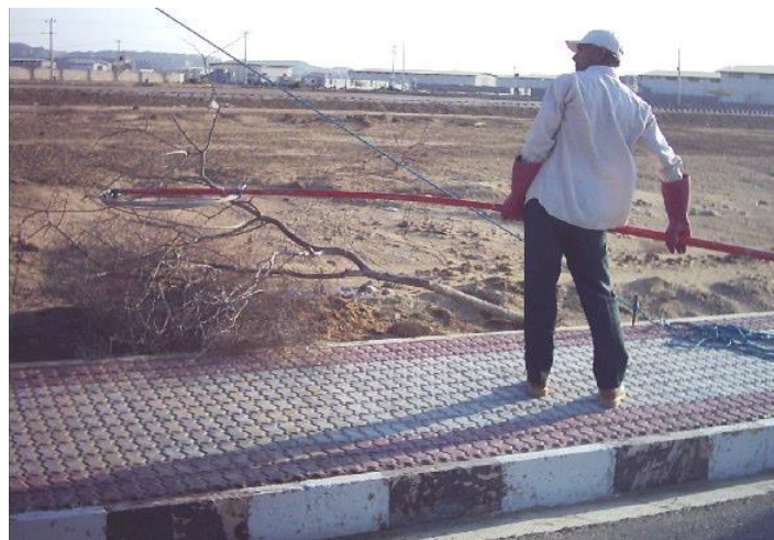
Fig 2.1: Dropping of conductor on earth [15]
