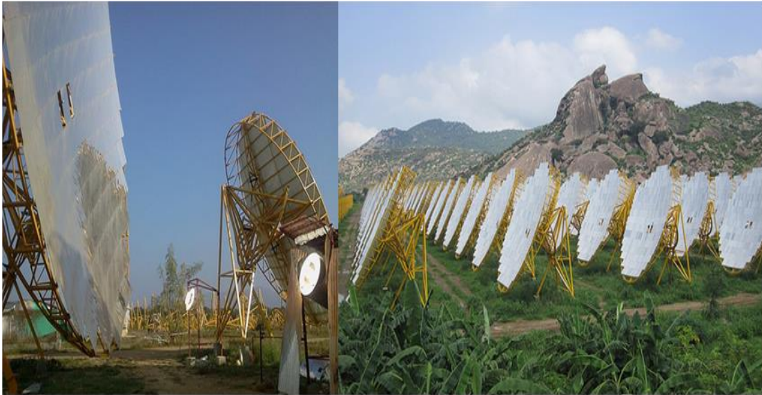
Figure 2.7 1 MW solar thermal power plant at Mount Abu, Rajasthan [44-45].
