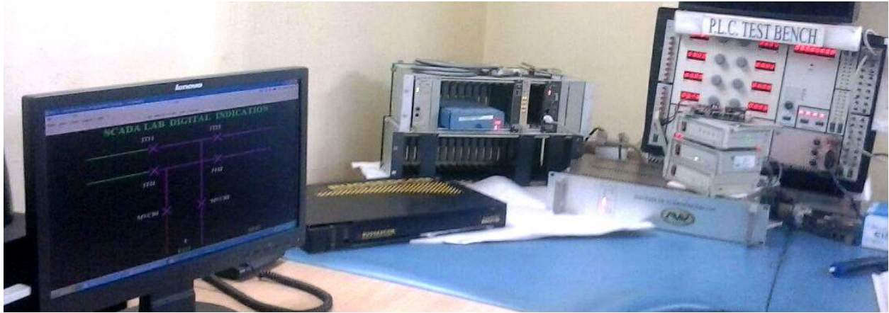
Fig.4.1: Test Setup to check/simulate SCADA message
